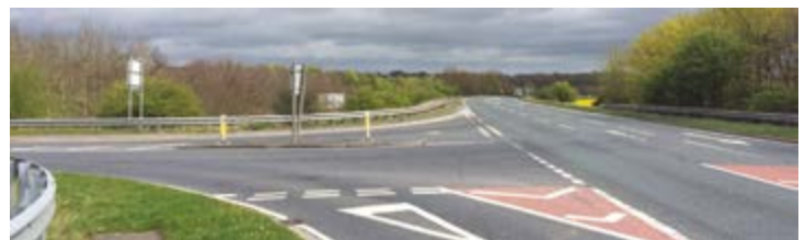
Existing A59 / York Road Junction
