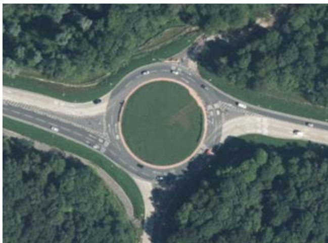
Existing A59 Roundabout
